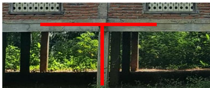
Figure 11. Pillars of the Godang House of the Pitopang Baghua Tribe
