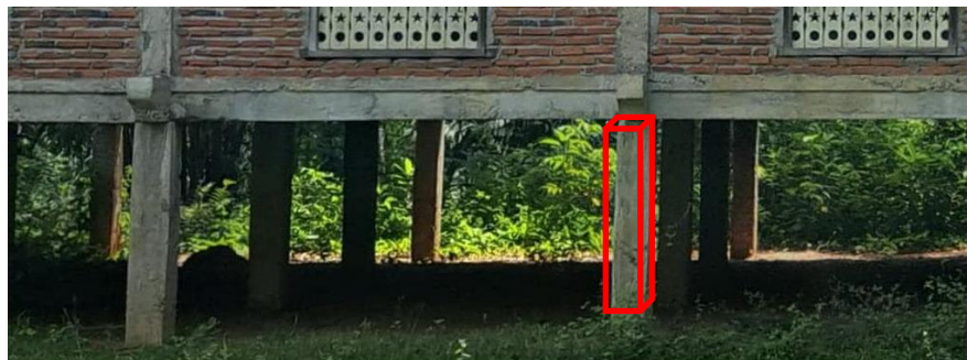
Figure 8. Pillar of the Godang House of the Pitopang Baghua Tribe
