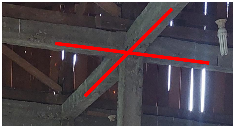
Figure 13. Ring Beam of the Godang House of the Pitopang Baghua Tribe
